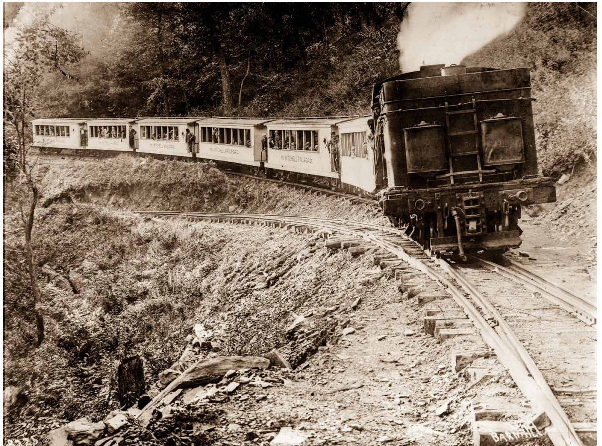
This photo shows the one of nine switchbacks used on this mountain line. Note the sharp downgrade on the left. All these cars are marked Mount Mitchell RR and the picture dates from 1921 when the line was operated for excursion only. (Mac Connery Collection)
