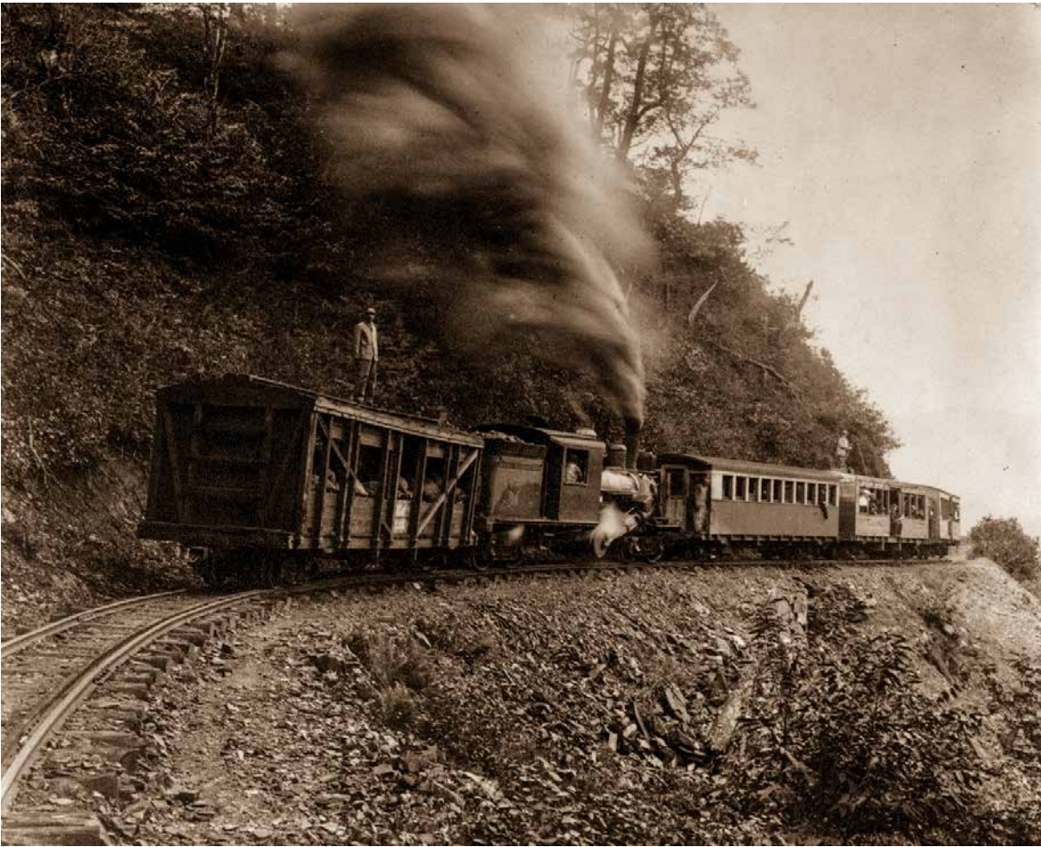
This photo shows the one of nine switchbacks used on this mountain line. Note the sharp downgrade on the left. All these cars are marked Mount Mitchell RR and the picture dates from 1921 when the line was operated for excursion only. (Mac Connery Collection)
