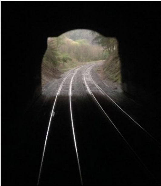
We are entering one of four tunnels on the Magnolia Cutoff. Note the notched sides that will allow "high containers" to go thru the tunnel. It also makes it look like a cats ears. Yes, Chessie the cat lives on...
