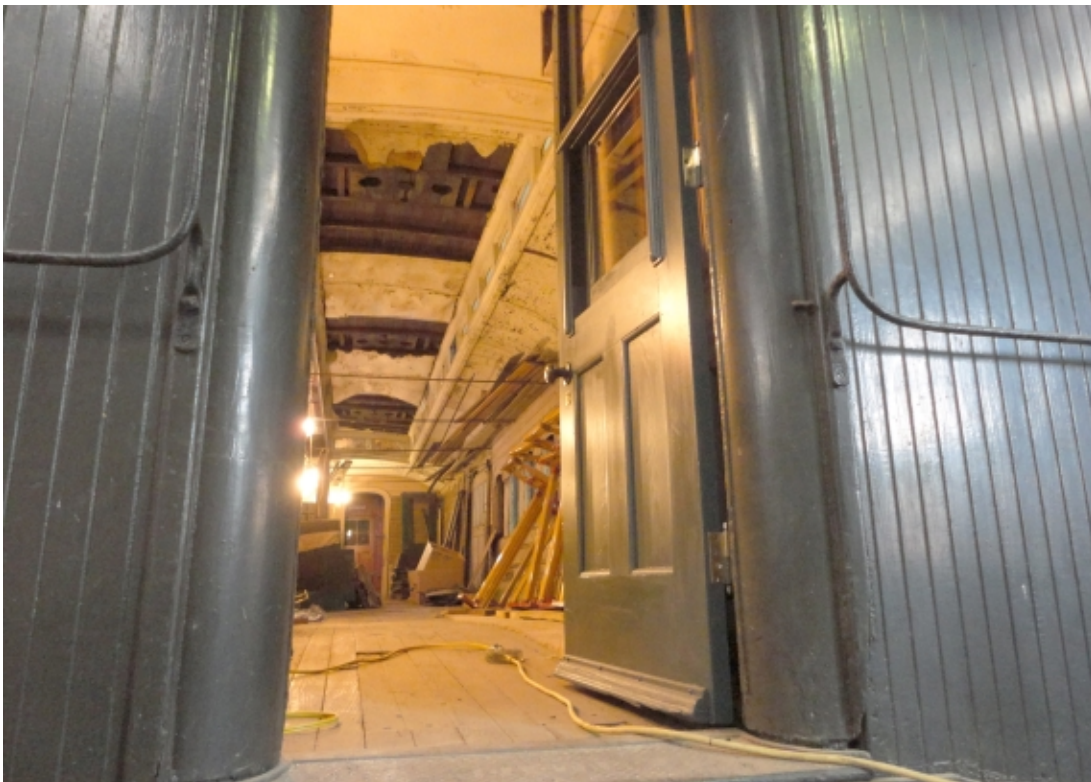
A wood passenger car being rebuilt at the M-CR.
