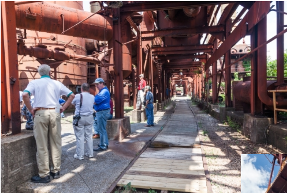
A view looking down the slag track which handled molten steel cars. If
