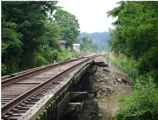
From the trestle – View to the Southwest toward Ecusta over the Davidson river near the community of Pisgah Forrest.
