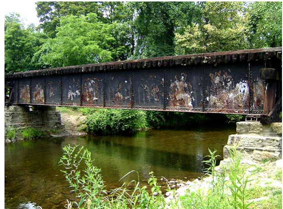
Road level view of the steel trestle over the Davidson River from Davidson River Road near the community of Pisgah Forrest .
