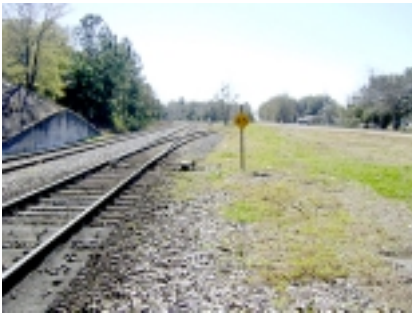
Switch SW to Gainesville in Waldo
